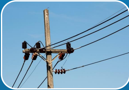
Overhead Power Lines
