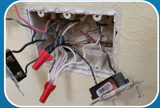
Exposed Conductors
